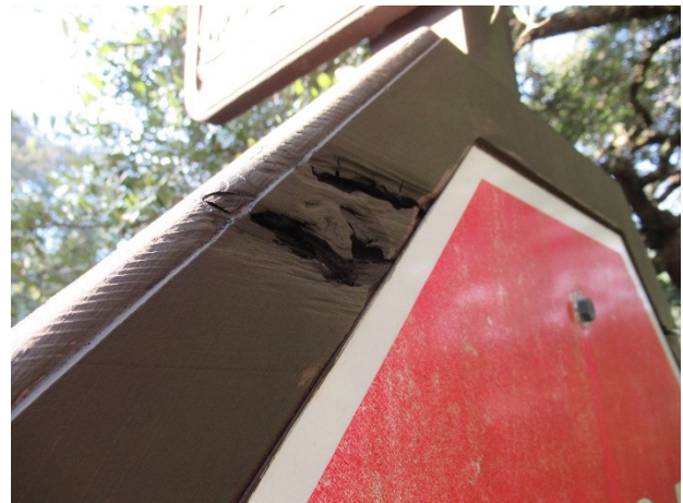
Street and traffic sign with wood rot and finish deterioration
