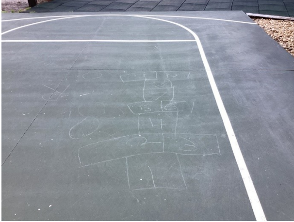
Basketball court overview
