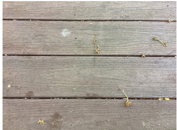
Deck boards fastened with screws
