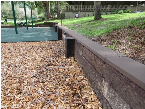
Playground retaining wall overview
