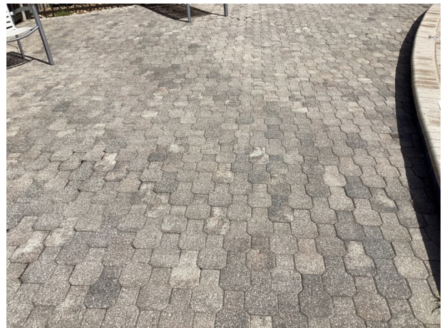
Paver pool deck overview
