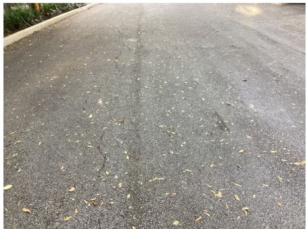
Pavement at clubhouse parking area
