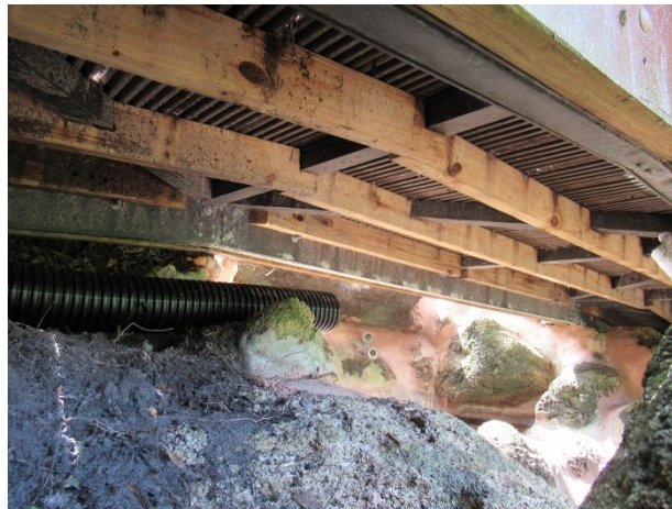
Pedestrian bridge underside
