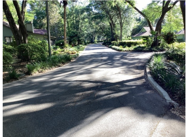
Pavement overview at Woodridge Trail
