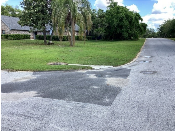
Pavement overview near English Brick Trail
