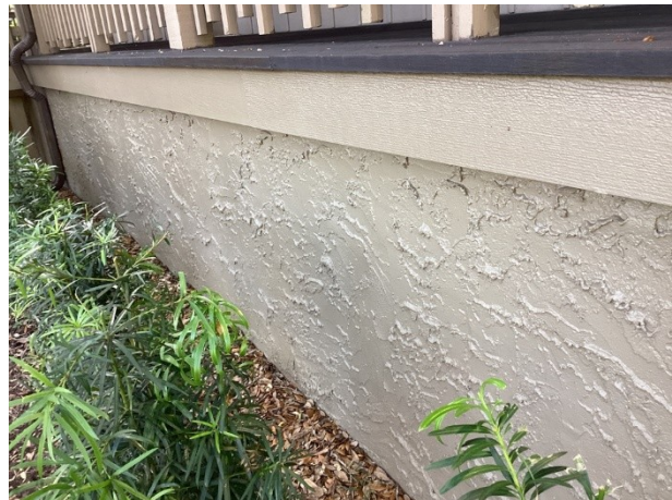
Stucco wall finishes
