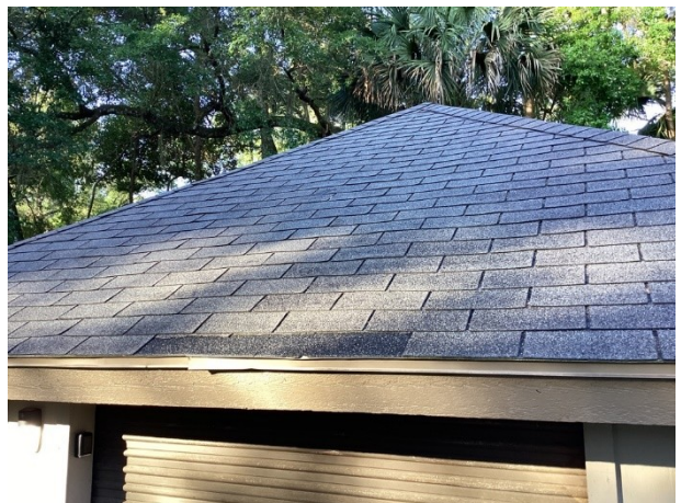
Storage building roof
