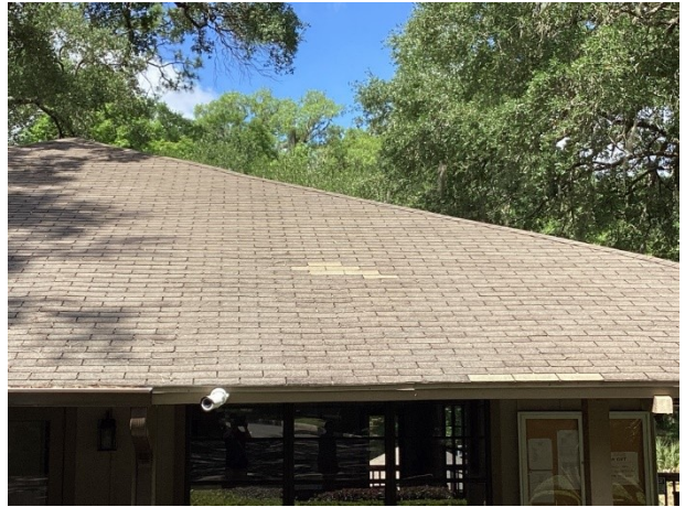
Roof repairs at clubhouse
