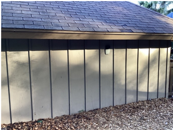
Wood siding at storage building
