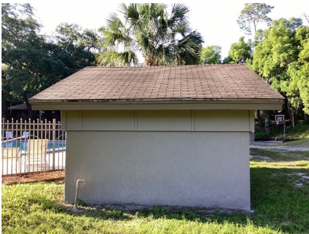
Pump house roof
