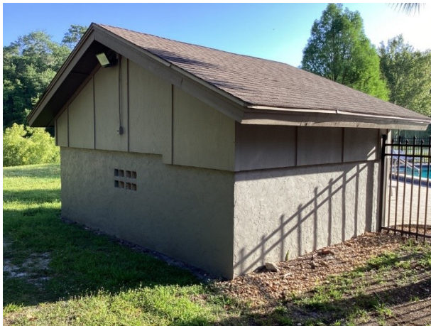
Pump house stucco and siding overview
