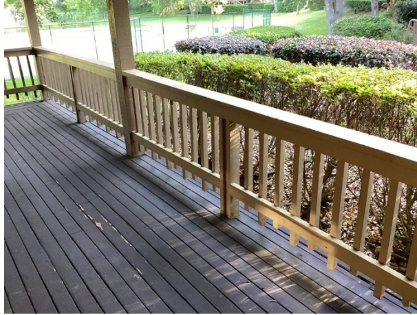
Railings at deck
