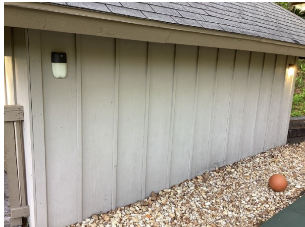
Wood siding at storage building
