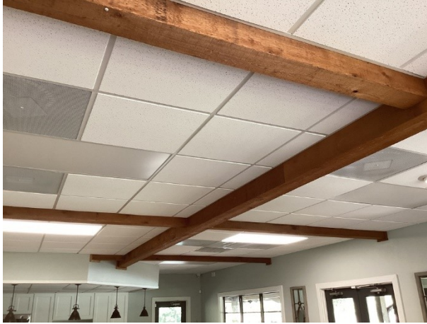
Acoustic ceiling tile overview
