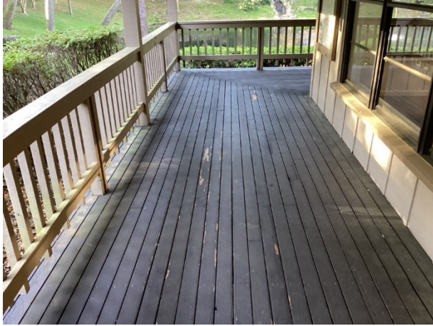
Clubhouse deck overview
