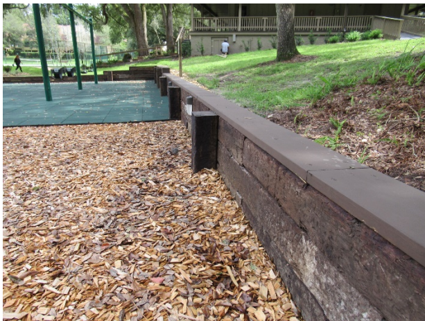
Playground retaining wall overview
