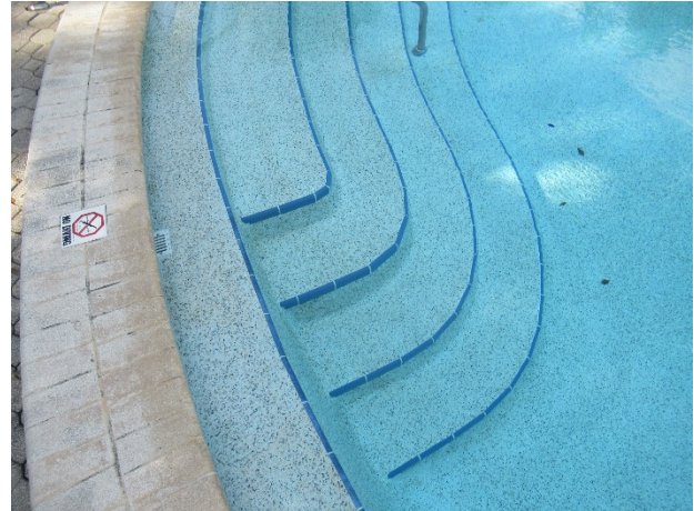
Plaster and tile finishes
