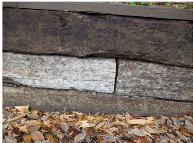
Playground retaining wall with weathered timber
