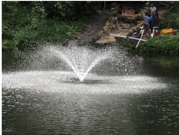
Pond Aerator overview
