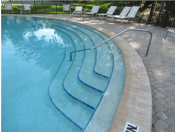
Plaster and tile finishes
