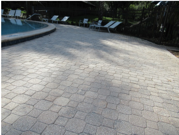
Pool deck overview
