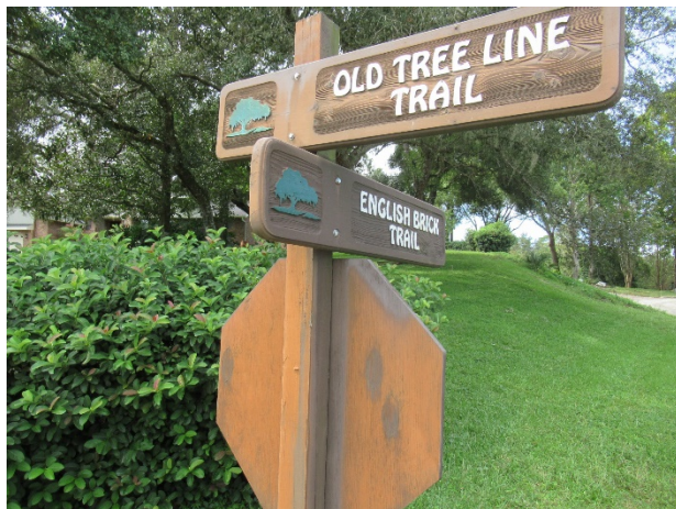
Street and traffic sign with finish deterioration
