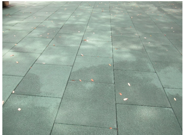
Safety surface overview
