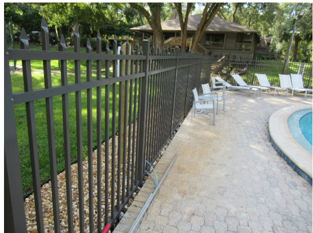
Aluminum fence overview
