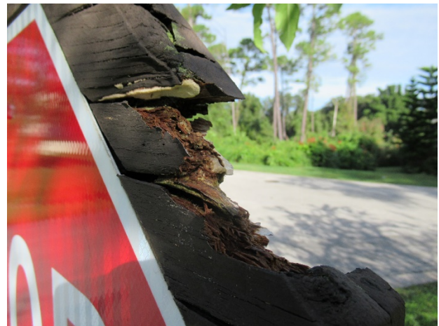
Street and traffic sign with wood rot
