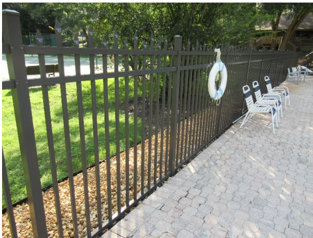
Aluminum fence overview
