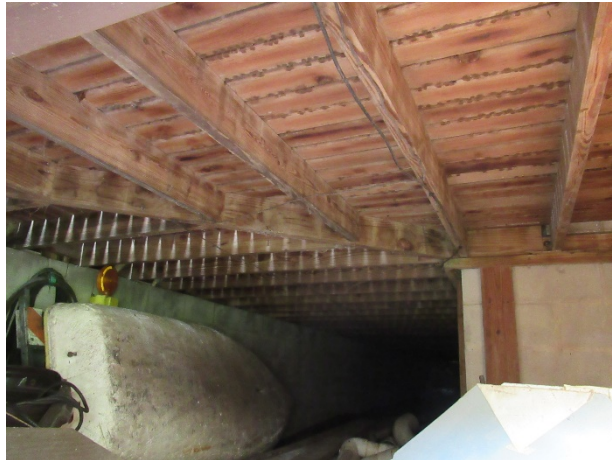
Wood deck underside
