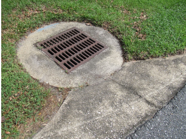
Catch basin overview
