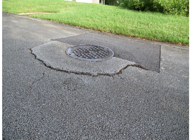
Asphalt Pavement – Sandy Bluff Trail
