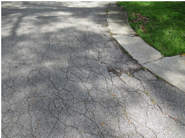
Asphalt Pavement – Secluded Oaks Trail
