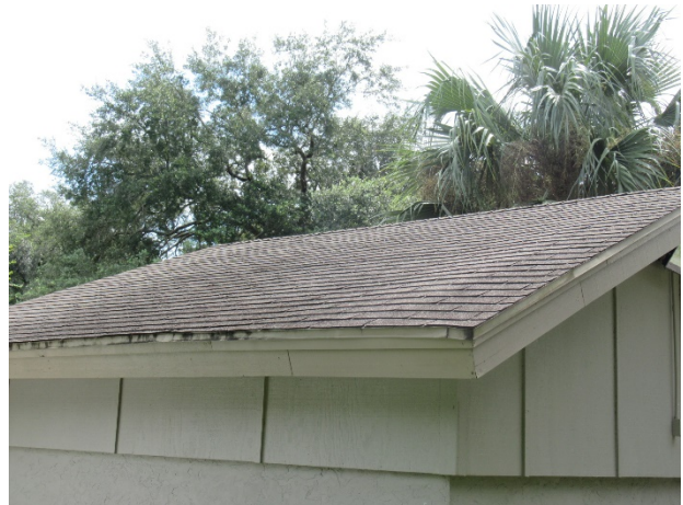
Pool mechanical building roof overview
