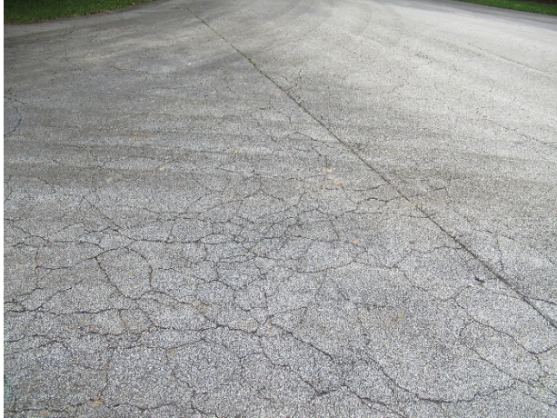
Asphalt Pavement – Fallen Timber Trail
