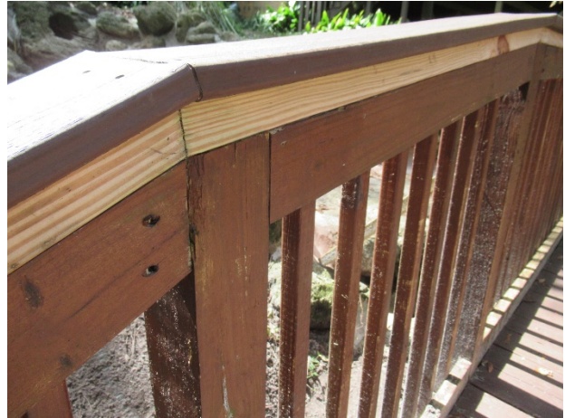
Pedestrian bridge railings
