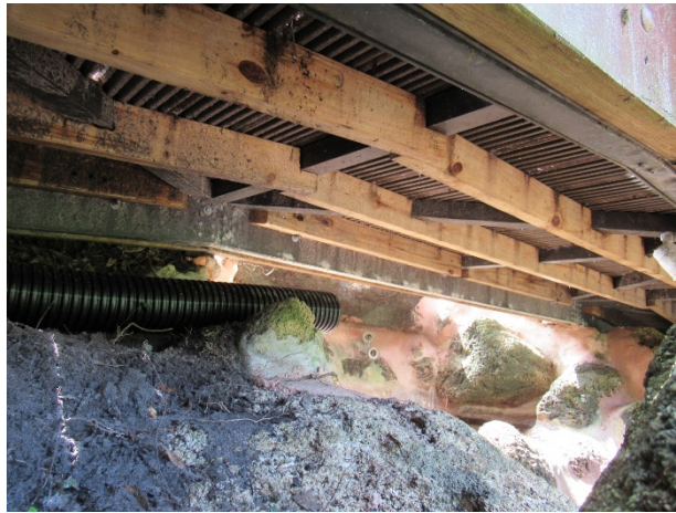
Pedestrian bridge underside
