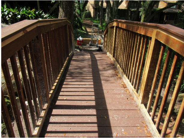
Pedestrian bridge overview
