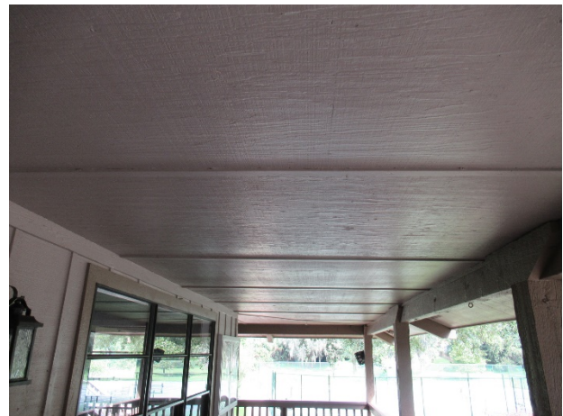
Wood soffit at clubhouse
