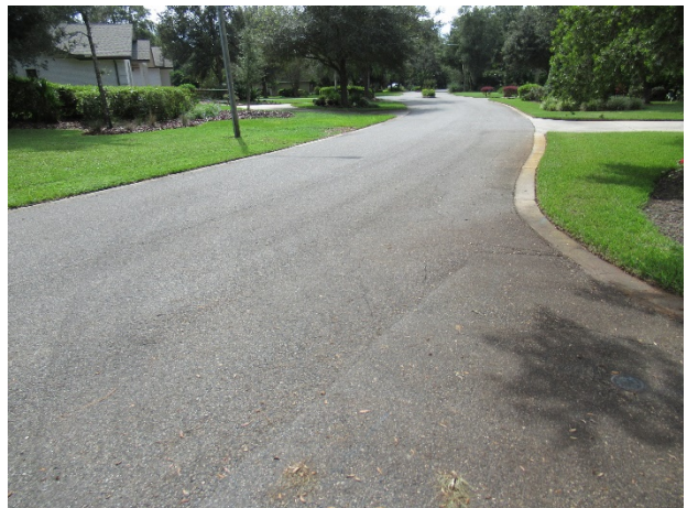
Asphalt Pavement – South Crooked Tree Trail
