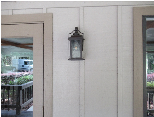
Siding and trim at clubhouse
