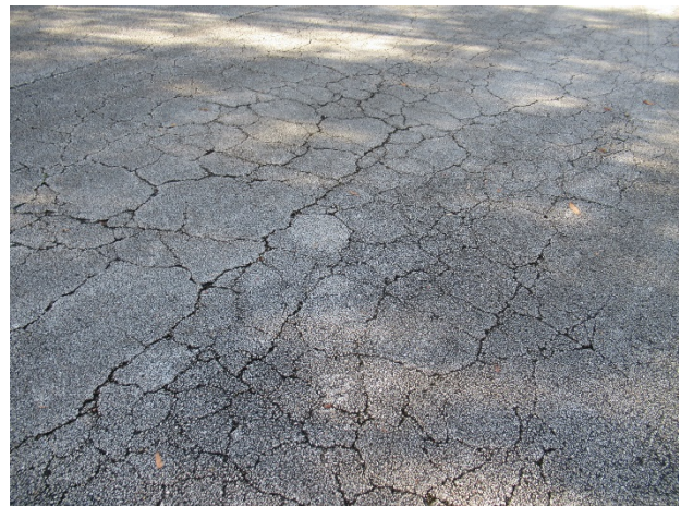
Asphalt pavement – Trail by The Lake
