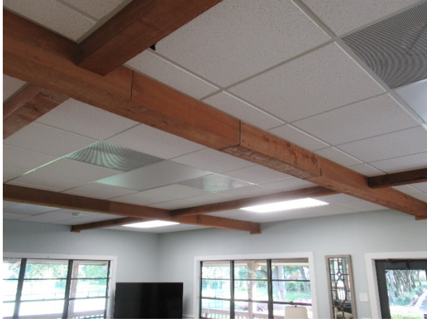
Acoustical ceiling tiles overview
