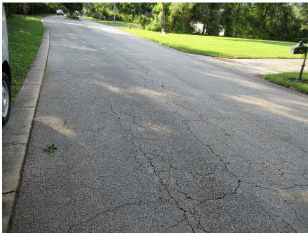
Asphalt pavement – north entrance
