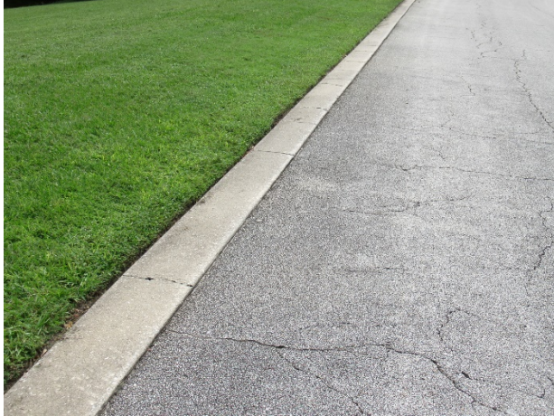
Ribbon curb overview
