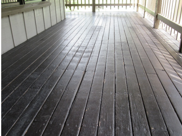
Wood deck overview
