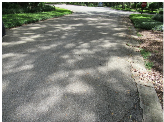
Asphalt Pavement – Lone Tree Trail
