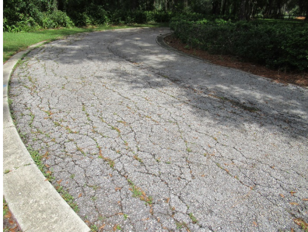
Asphalt Pavement – Shady Branch Trail
