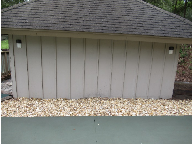
Siding at maintenance shed
