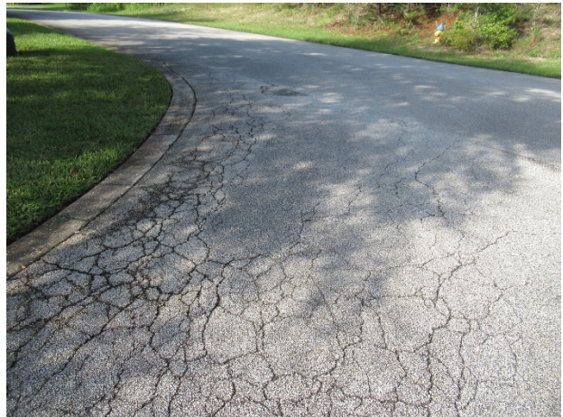
Asphalt Pavement – Sandy Bluff Trail
