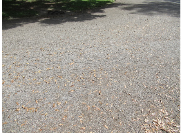
Asphalt Pavement – Shady Branch Trail
