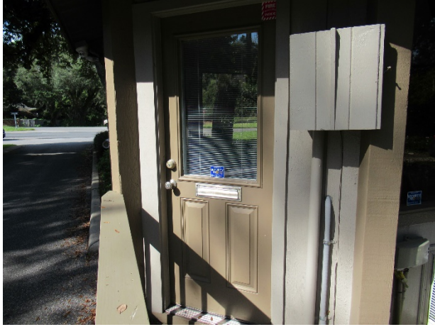
Door at office
