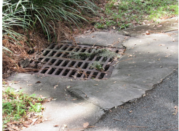
Catch basin overview
