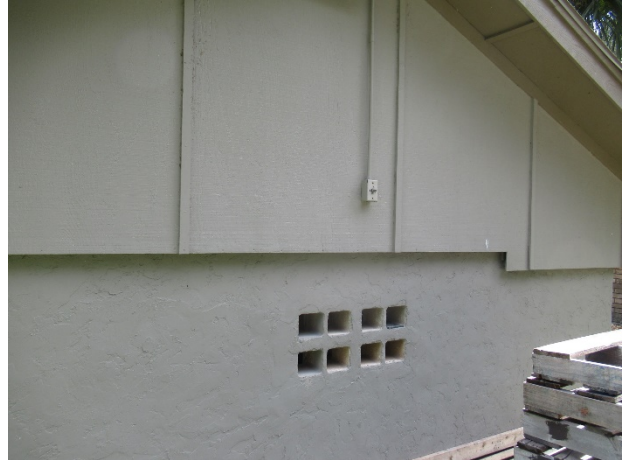
Siding at pool mechanical building
