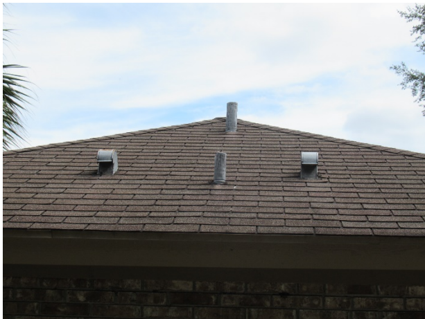
Pool rest room building roof overview
