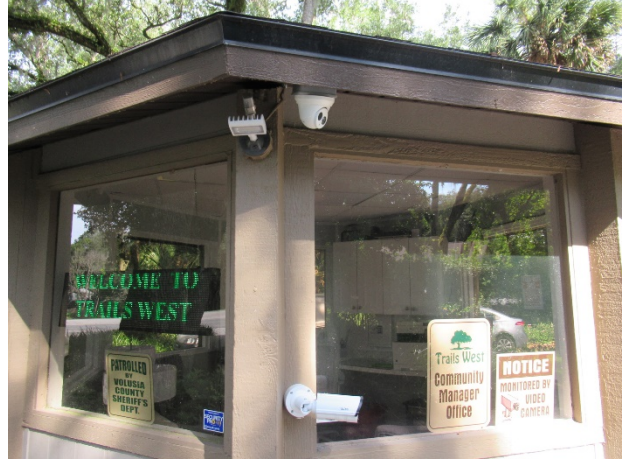
Windows at office
